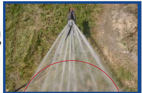
The red line in the photo depicts the point in which the jets of the nozzle come in contact with the floor of the pipe creating the "water shovel" affect.
