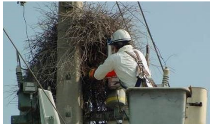
Figure 5. Removal of monk parakeet nests from electric utility distribution poles is a short-term solution as birds quickly rebuild.
